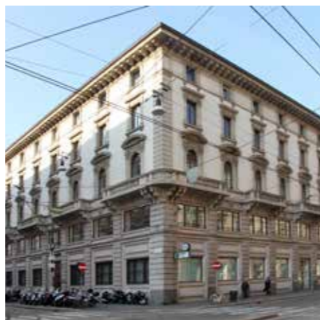
Offices Cantù-Orefici Client: Savills Investement Management Preliminary design, definitive design, executive and art direction. Milan 2017/On going Built surface: 12.000 m 2
