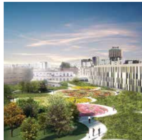
Ospedale Maggiore Policlinico International competition, winner Site demolition Client: Fondazione IRCCS Cà Granda Milan 2007 / ongoing Preliminary design, definitive design and artistic direction Project area: 80.000 m 2 ; built surface: 70.000 m 2
