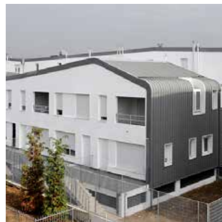
Social Housing Seregno Task completed, carried out project Client: Comune di Seregno Seregno, Milan 2004 / 2006 Preliminary design, definitive design, construction design Built surface: 2.700 m 2
