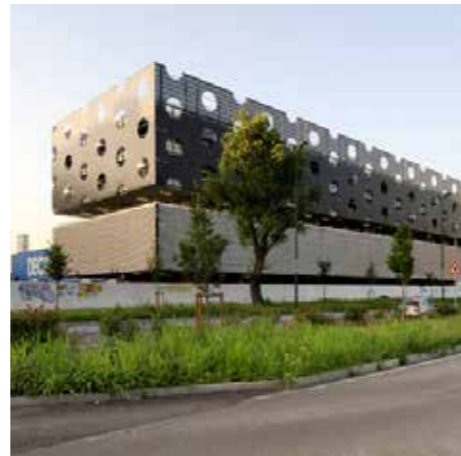
Shopping center Task completed, carried out project Client: F.I.L.Casa Service S.r.l. Cinisello Balsamo-Sesto San Giovanni (Mi) 2001/2011 Preliminary design, definitive design, construction design, works supervision Built surface: 12.500 m 2 - extension: 1.700 m 2 Photo credits: Paolo Rosselli
