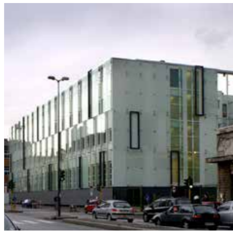
Bicocca building 307 Task completed, carried out project Client: PRELIOS S.p.A. (ex Pirelli & C Real Estate) Milan 2003 / 2005 Preliminary design, definitive design and construction design, AD Built surface: 10.000 m 2 Photo credits: Paolo Rosselli
