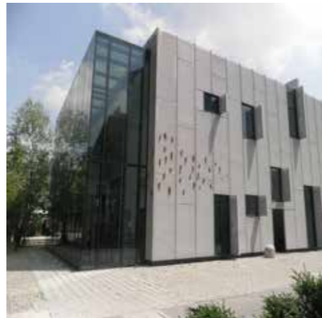
Arts incubator Task completed, carried out project Client: Hines Italia Sgr Milan 2006 / 2011 Preliminary design, definitive design, construction design and artistic direction Built surface: 2.000 m 2
