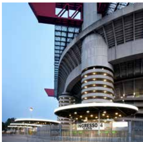
Stadio San Siro task completed, carried out project New gates of access and new Inter change areas Schematic design, definitive design, construction design and artistic direction Client: Consorzio Milan Inter Milan 2004 / 2005
