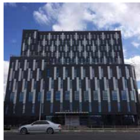
Hotel Misheel EXPO Under Construction Client : Termigas Bergamo S.p.A. Ulaanbaatar, Mongolia 2014 / ongoing Preliminary design and definitive design Built surface: 17.500 m 2
