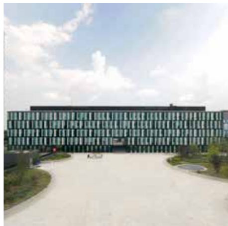
RCS - Mediagroup building B5 Task completed, carried out project Client: Iniziativa Immobiliare Due s.r.l. (Prelios S.p.A. - Morgan Stanley - RCS Mediagroup) Milan 2008 / 2011 Preliminary design, definitive design and construction design, artistic direction Built surface: 12.500 m 2 Photo credits: Paolo Rosselli
