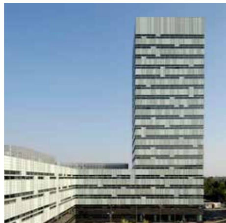
RCS - Mediagroup building C Task completed, carried out project Client: Iniziativa Immobiliare Due s.r.l. (Prelios S.p.A. - Morgan Stanley - RCS Mediagroup) Milan 2003 / 2010 Preliminary design, definitive design and construction design, artistic direction Built surface: C, 25.000 m 2 Photo credits: Paolo Rosselli
